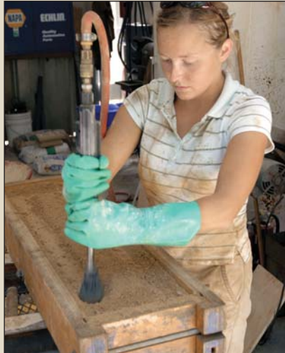
Using a pneumatic ram, Haley Mills tamps the coquina, sand, and cement mixture into Wright's original molds. A key to the performance of the blocks is a graded aggregate — a range of sand particles that allows for denser packing, ultimately leading to a more impervious block.
